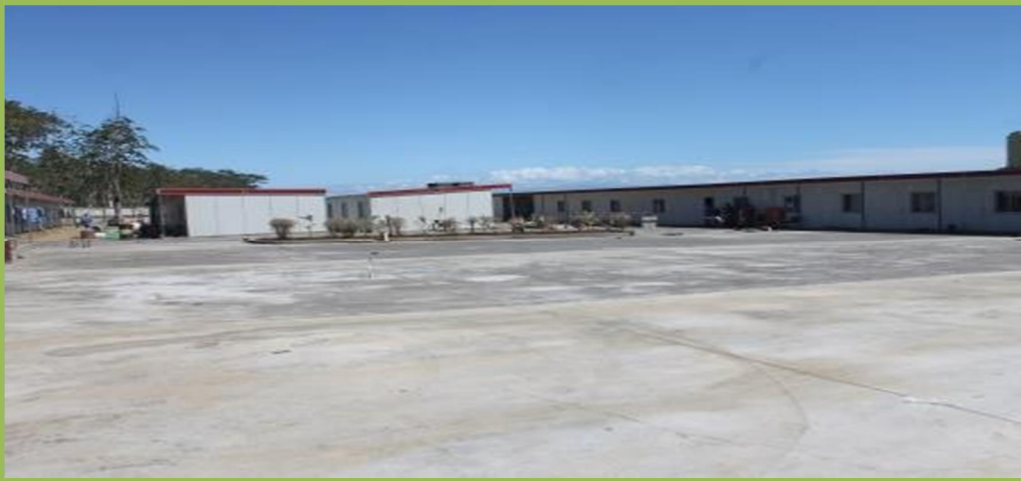
Figure 5: SCG accommodation and office supply site
