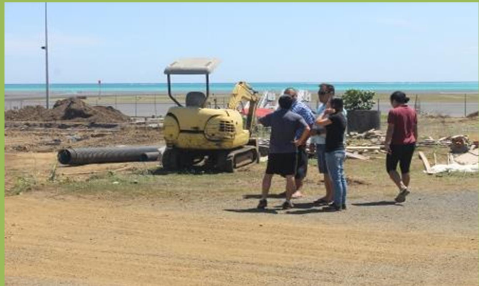
Figure 6: Construction site East section of airport
